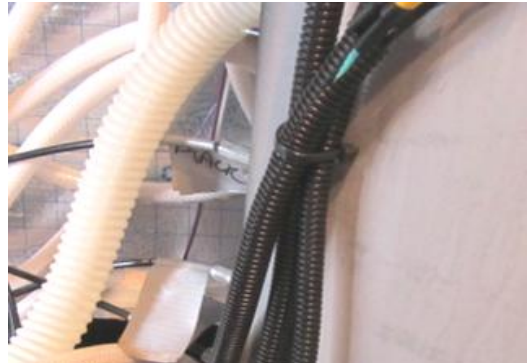
Fig. 18 A IP 66 wire pairs and 12V supply wires sheathed over and tie wrapped
