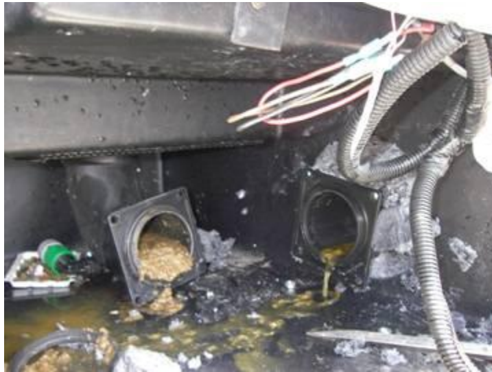
After Removing Valves and Manifold
